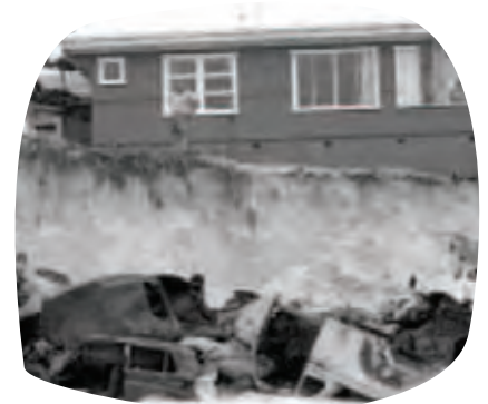
Car bodies used to try and stop the progress of erosion on the Gold Coast, 1967.
