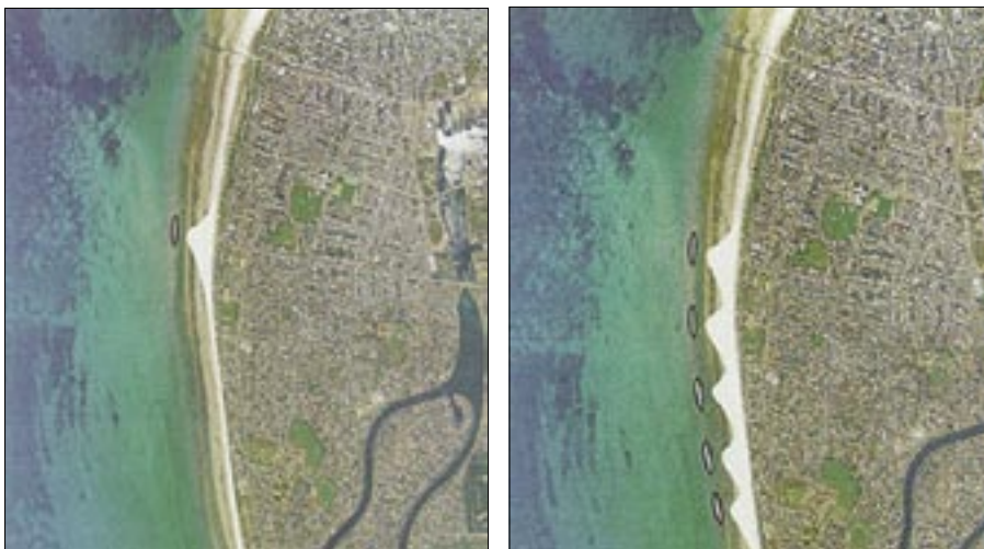
Figure 4.5 Aerial photographs illustrating the stages of the Semaphore Park Coast Protection Strategy (a) Stages 1 and 2 (b) Stage 3
