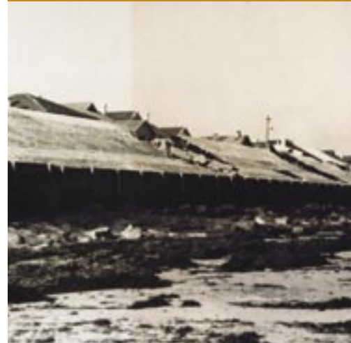
Early photo of seawall sand impoundment that prevented dune erosion at Henley Beach
