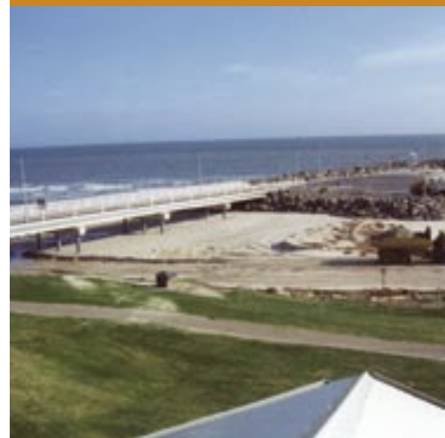
Adelaide Shores boat haven overpass
