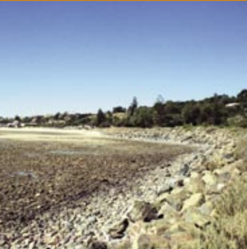
Rip-rap seawall at Seacliff, 2004
