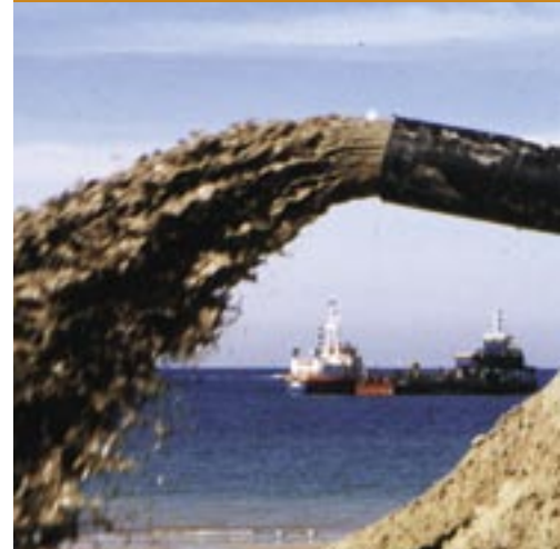
Brighton beach replenishment via dredging offshore from Port Stanvac
