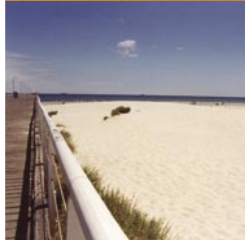
Build-up of sand at the Semaphore jetty
