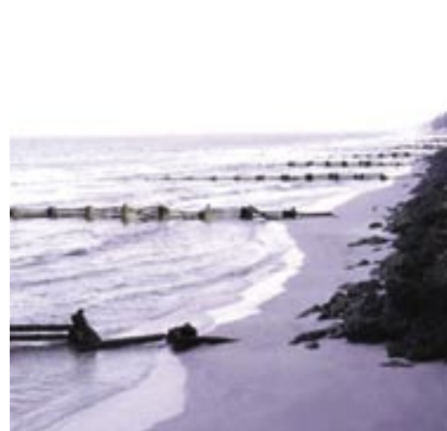
Groynes and seawall in Florida, USA (US Geological Survey)
