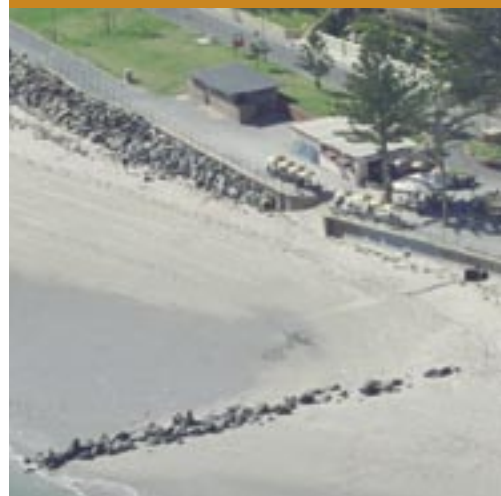
Rock groyne at the Broadway, Glenelg
