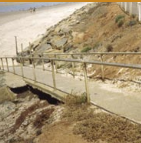
Beach access – ramp in a seawall
