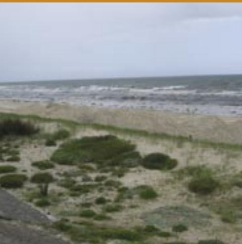
Placing sand north of the Torrens Outlet, November 2004 (City of Charles Sturt)
