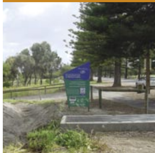
Foreshore stormwater outlet at Taperoo
